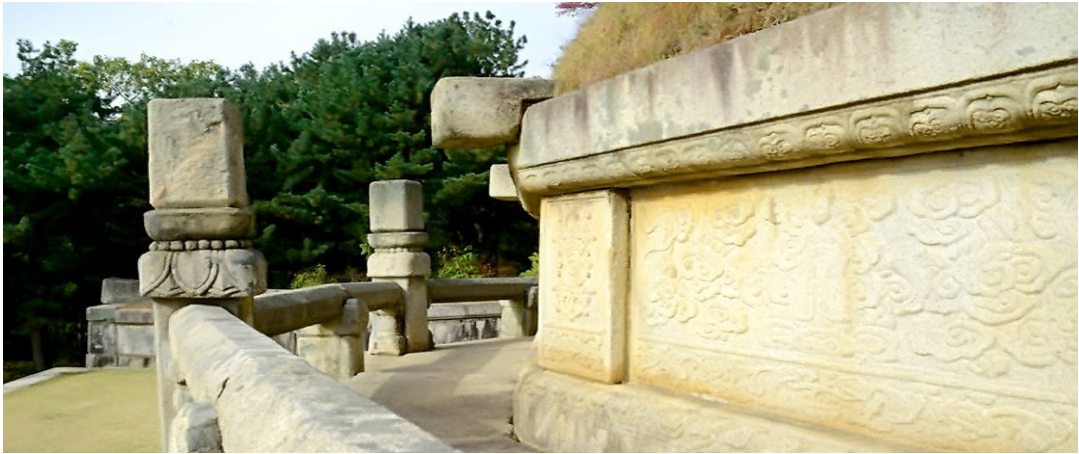
Folding screens and stone rails are neatly dovetailed.
