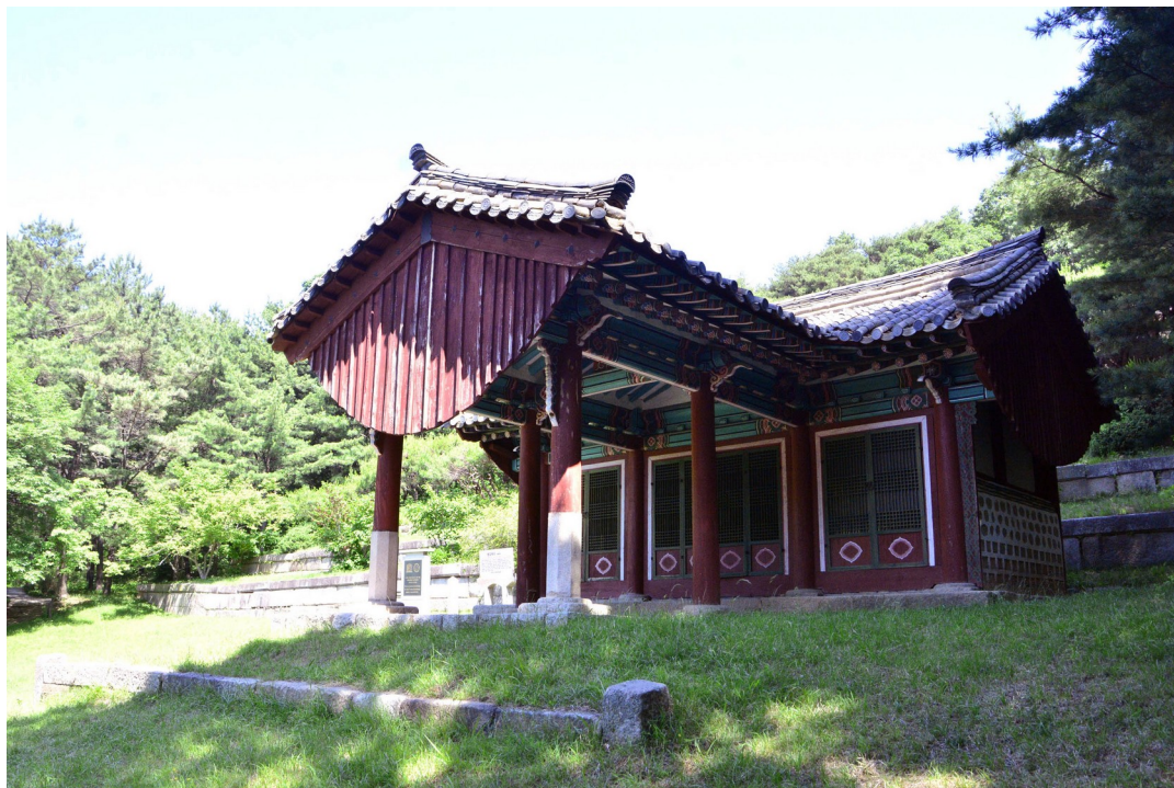
Building for memorial service and its colourfully-painted interior
