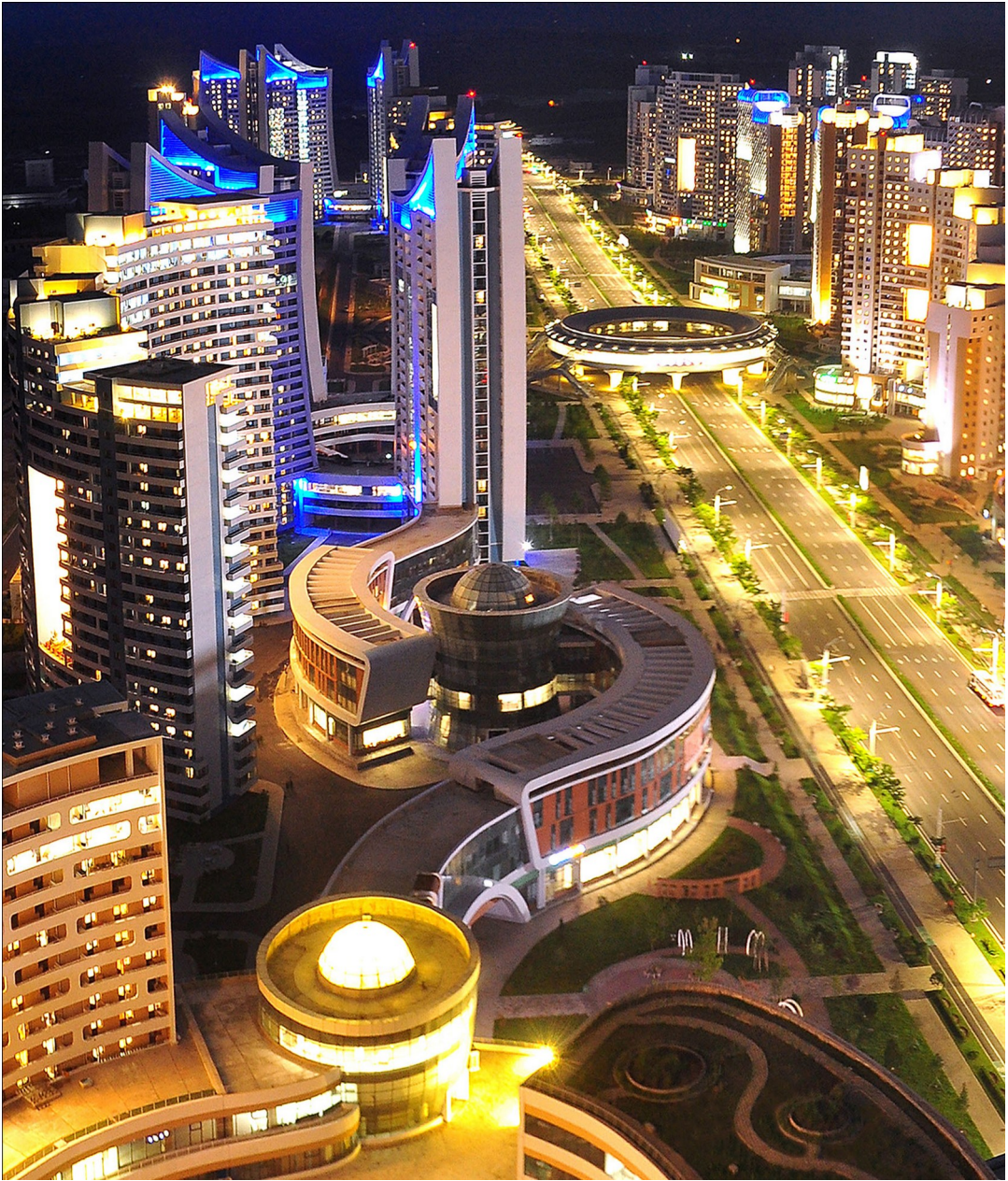
Part of 10 000 flats in Songhwa Street built only in a year pursuant to the construction plan of 50 000 flats in Pyongyang (2022)
