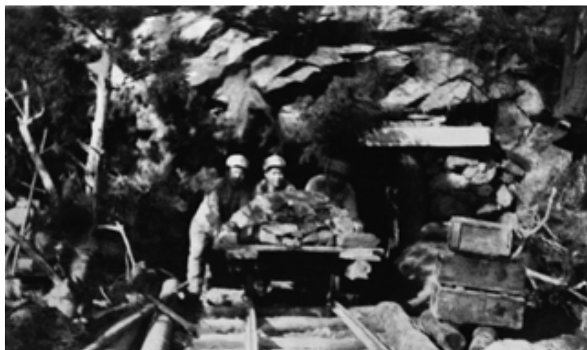
The KPA soldiers dig a tunnel.
