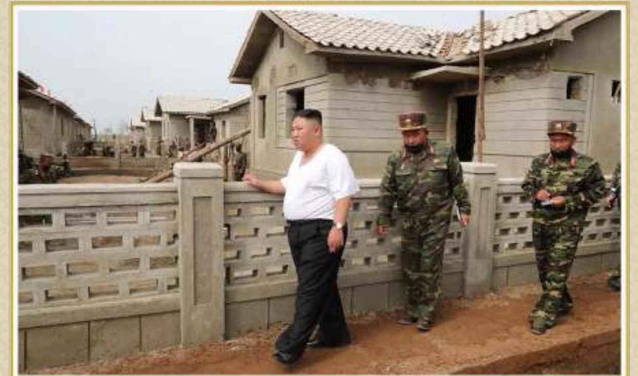
Kim Jong Un gives on-site guidance over construction in the flood-hit Taechong-ri area, Unpha County, North Hwanghae Province, in September Juche 109 (2020).
