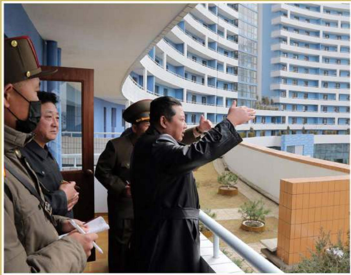
Kim Jong Un gives on-site guidance at the construction site of 10 000 flats in the Songsin and Songhwa areas nearing completion in March Juche 111 (2022).
