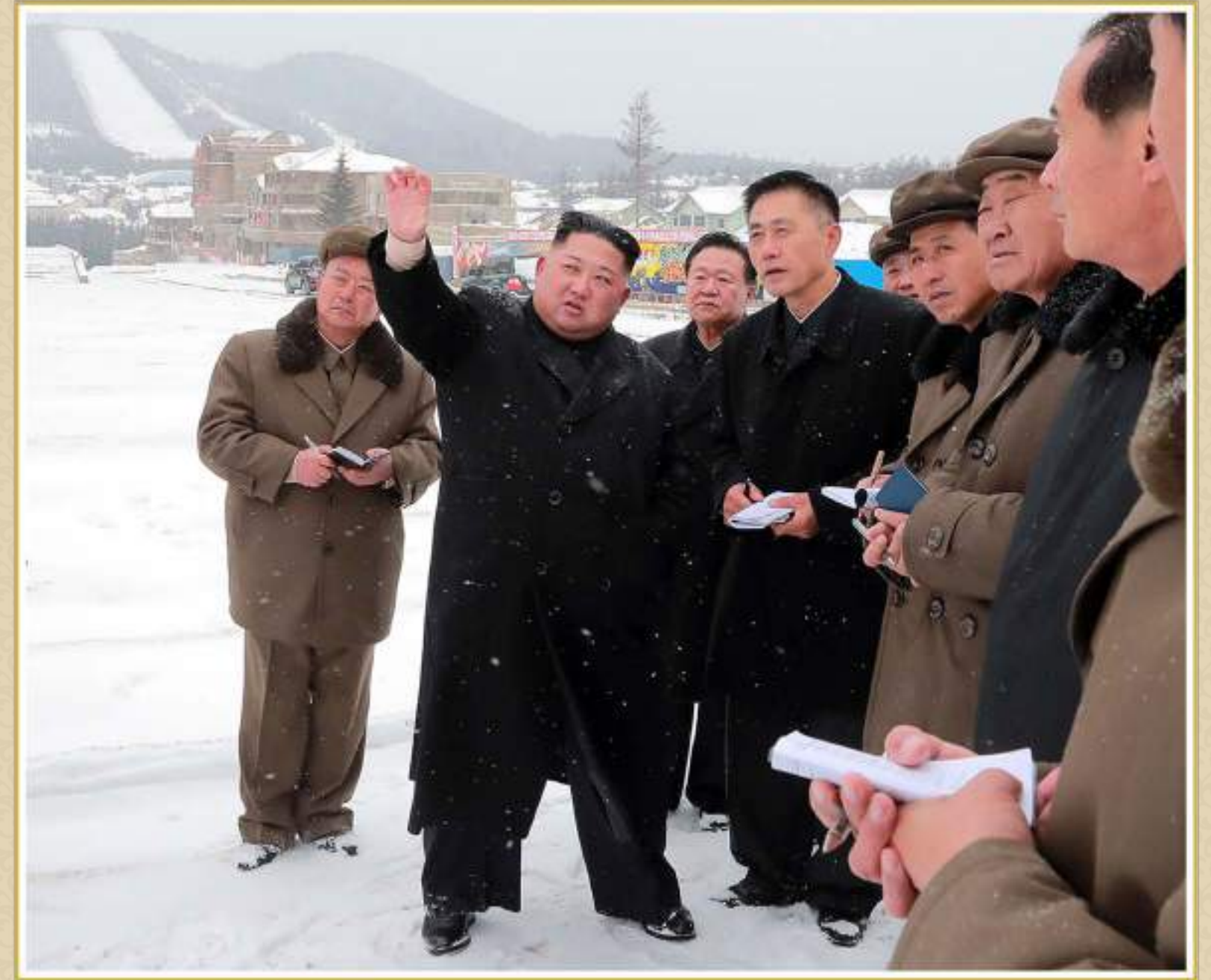
Kim Jong Un acquaints himself with the construction of the Samjiyon County town in October Juche 107 (2018).
