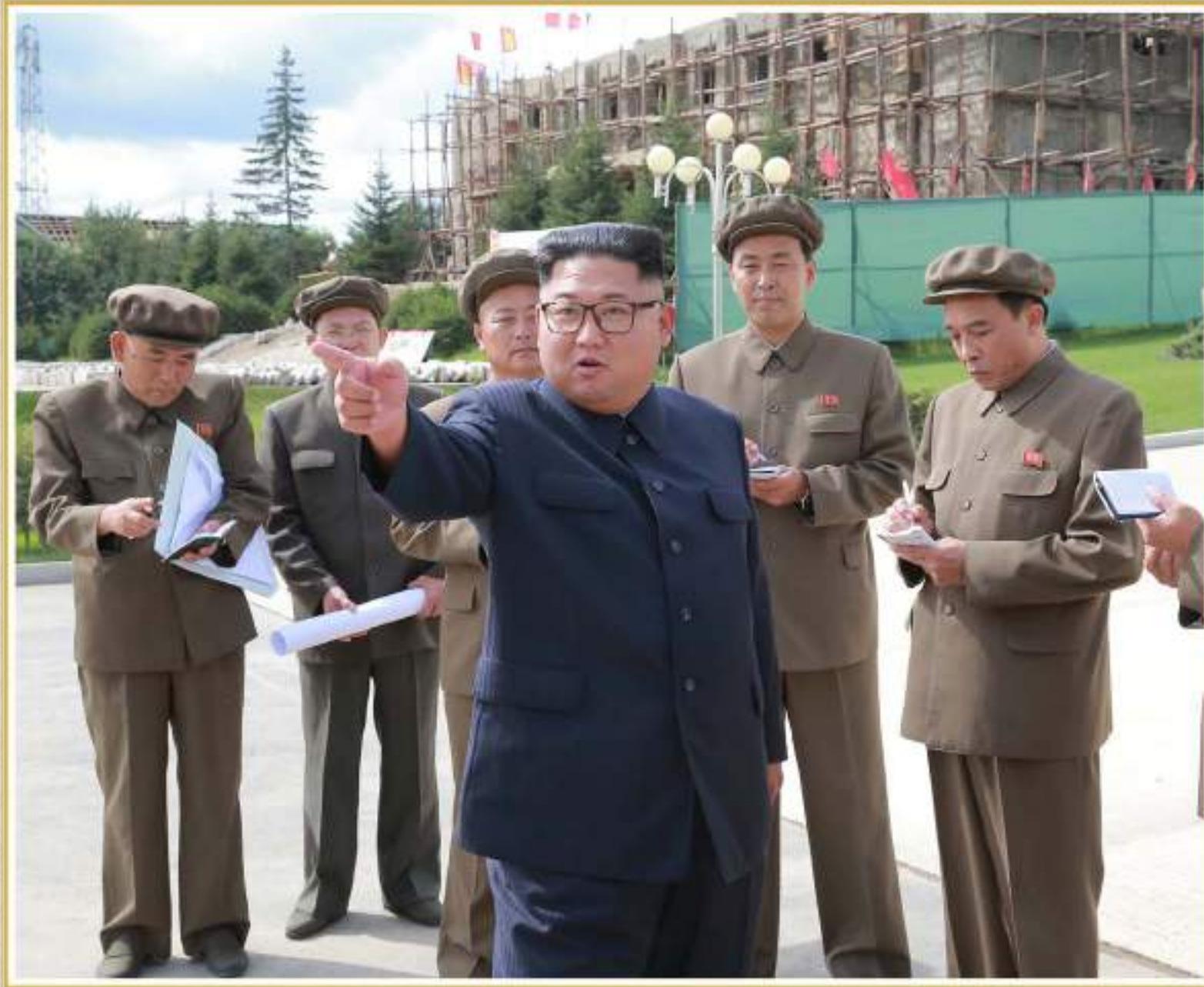
Kim Jong Un gives on-site guidance at construction sites in Samjiyon County again in August Juche 107 (2018).
